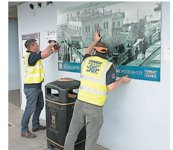
The installation of the Marine Spa graphic by Torbay Direct printers.
