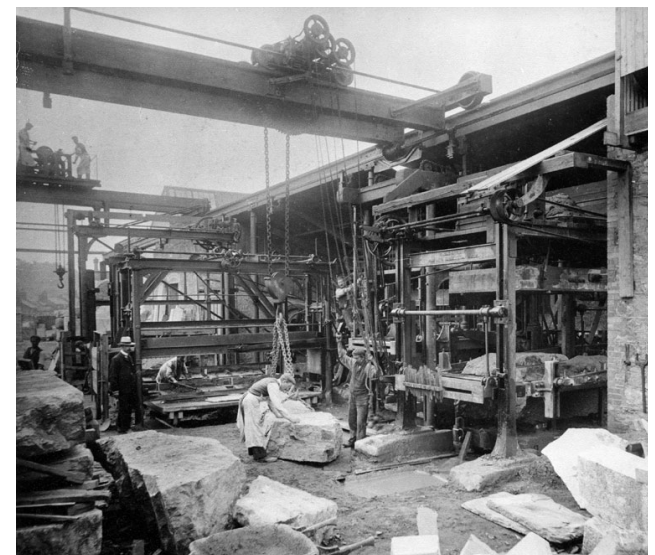
Jenkins Marble Works (PR4468)
